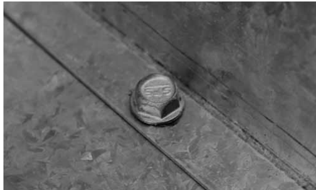
Figure 1.12.3: SIDE SEAM SELF-DRILLING SCREW
