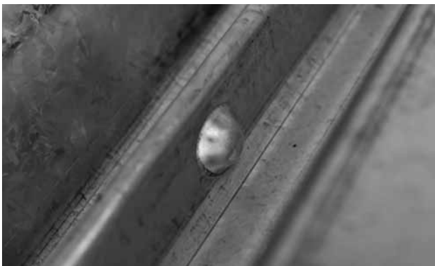
Figure 1.12.2: BUTTON PUNCH SIDE LAPS
